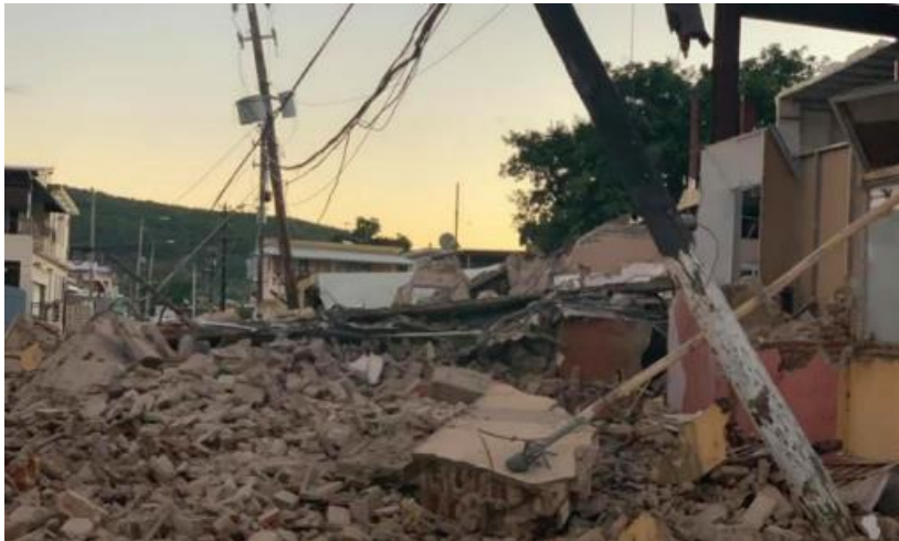
Building and power infrastructure damage, Guanica, Puerto Rico
